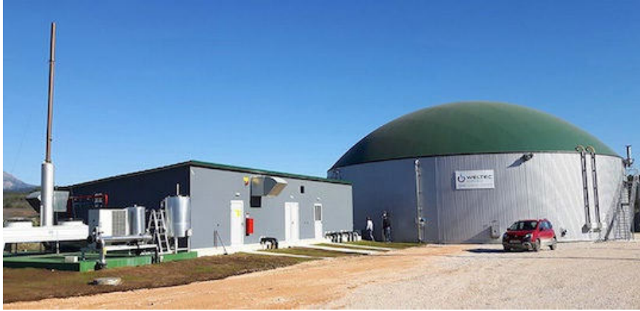
Figure 8 Anaerobic digester for the fermentation of manure into compost and biogas
