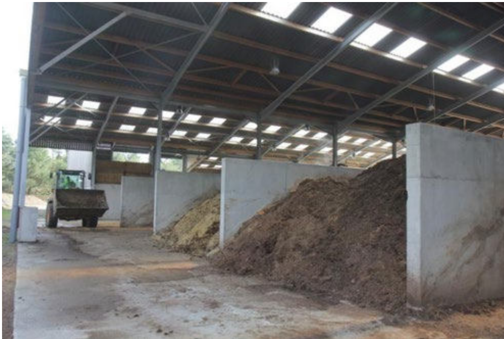
Photos 3 Closed composting platform where gas emissions can easily be captured and cleaned
